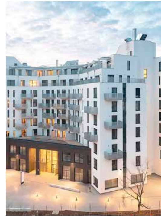
Althan Park Residential Complex | Austria
